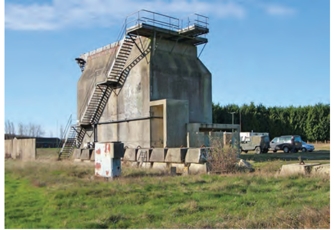
K1 stand used to test vertical rocket motors
